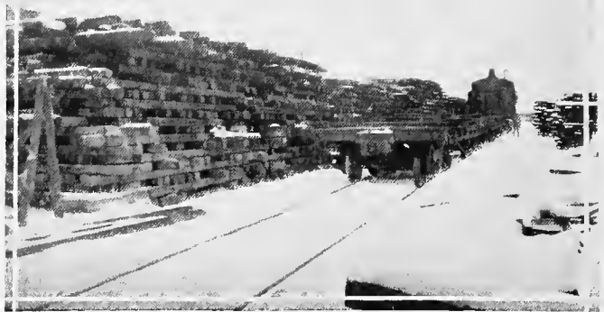
Storage of Steel Billets in Steel Yard for 155 mm. Shell Forgings
